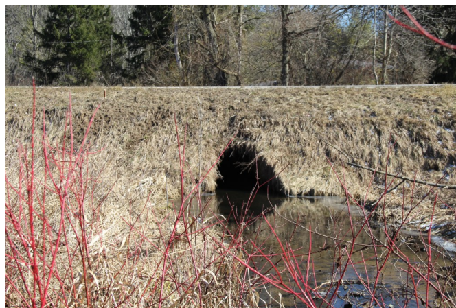
The undersized Maple Island Road culvert which backs-up the Maple River during high flows.
