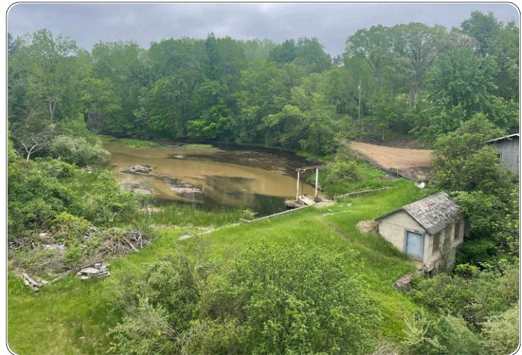
The large hydraulic drop of the structure, naturally steep stream slope, and over a century of sediment build up present many technical challenges to restoration. MRWA is raising \$1.1 million for dam removal and habitat restoration. The project is in the Engineering and design phase, and fundraising currently underway. Construction is expected to begin in summer of 2026.
